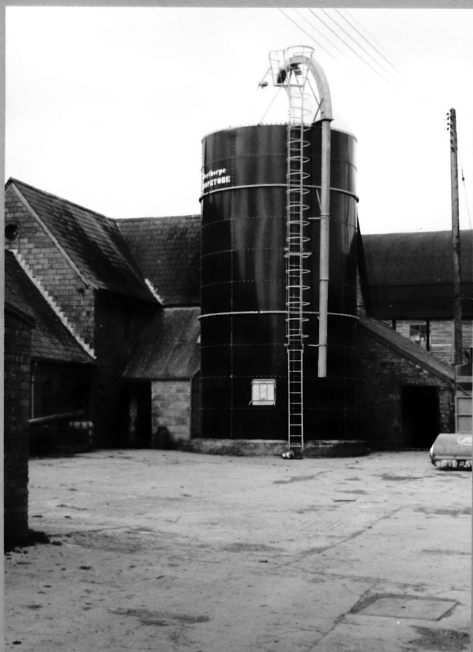
- and, in the yard below the farmhouse, the silo from the top of which the photographs were taken.
